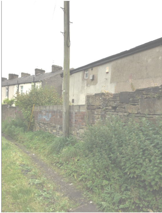
Rear of the property from the back street
